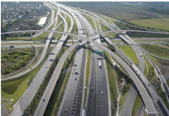
I-595 Corridor Roadway Improvement
